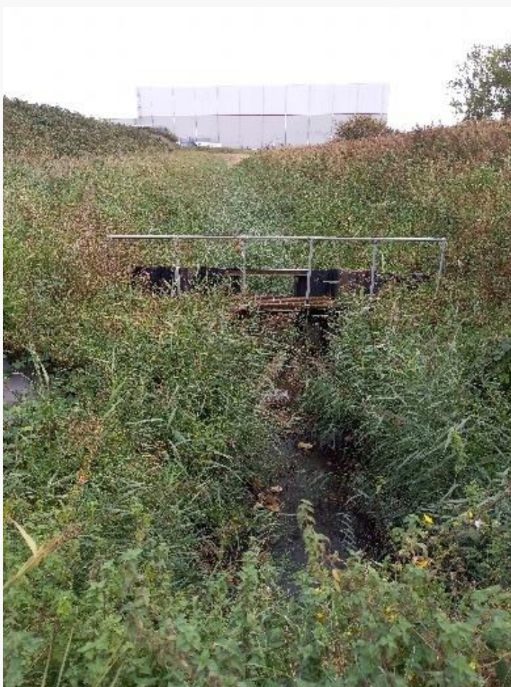
TF 45455 07895 View of IDB adopted drain (facing East), which bisects the EfW CHP Facility, (between nodes 33 and 45). Image captured from the culverted section, which provides vehicular access between the north and south sections of the site. Note the DFDS Logistics Warehouse in the distance.
